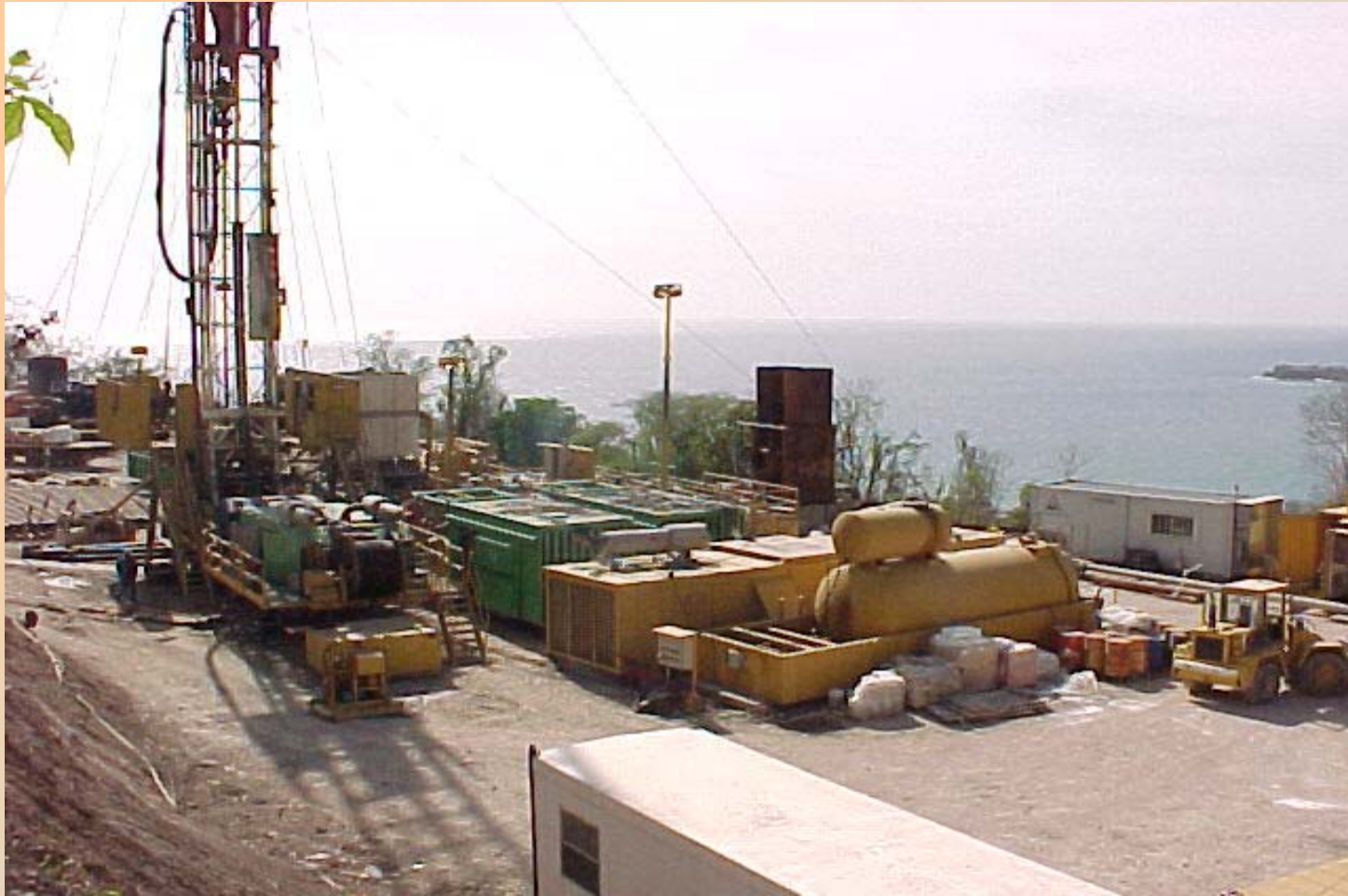
The well platform and the equipment used for drilling directional wells BO-5, BO-6 and BO-7 (Dec. 2000 - May 2001). The Caribbean sea in background
