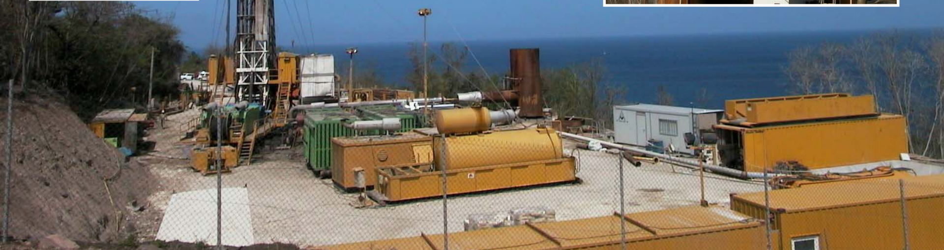
View of the well pad for drilling operations of the three new wells- BO-5, BO-6 et BO-7- in Bouillante. Above (left), details of the BO6 wellhead and above (right) vapor discharge during a production test (May 2001)
