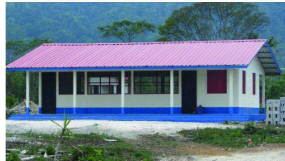
Residents will benefit from a new school in the Santa Rosa Community Resettlement in the Adjacency Zone. Below: Sergio Benítez, Director of the Office of the General Secretariat in the Adjacency Zone, carries out a verification with the help of GPS equipment
