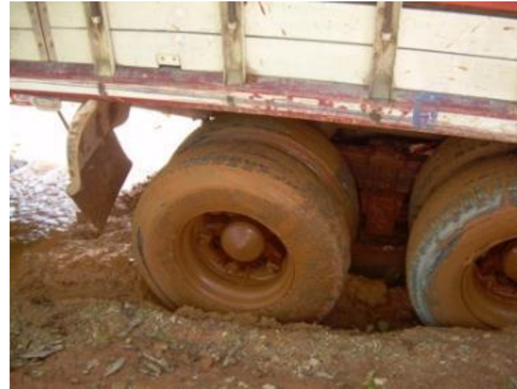
Poor road conditions and inaccessible areas
